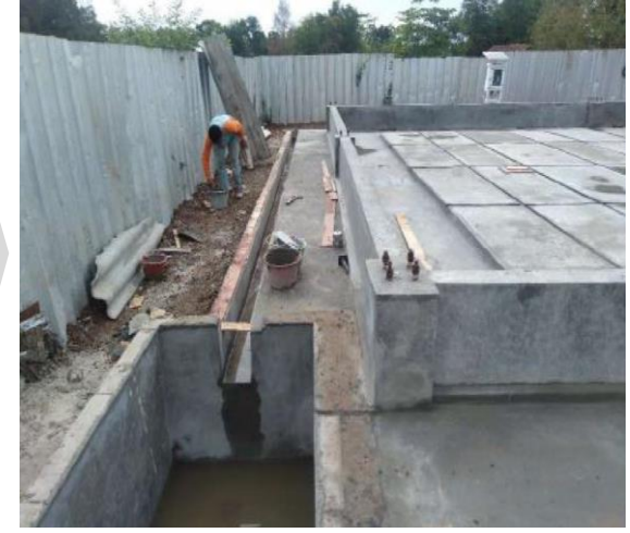
Floor construction of the membrane filter area
