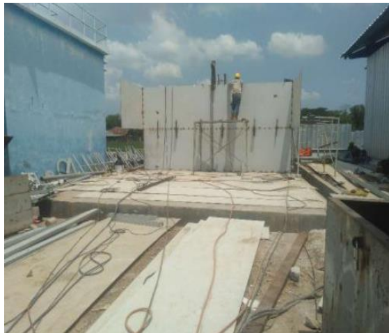
Sedimentation tank installation
