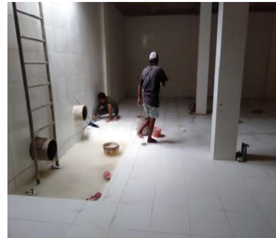
Finish laying tiles inside plant
