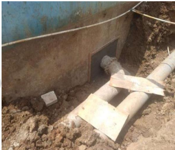
Connect pipes from the existing purification plant
