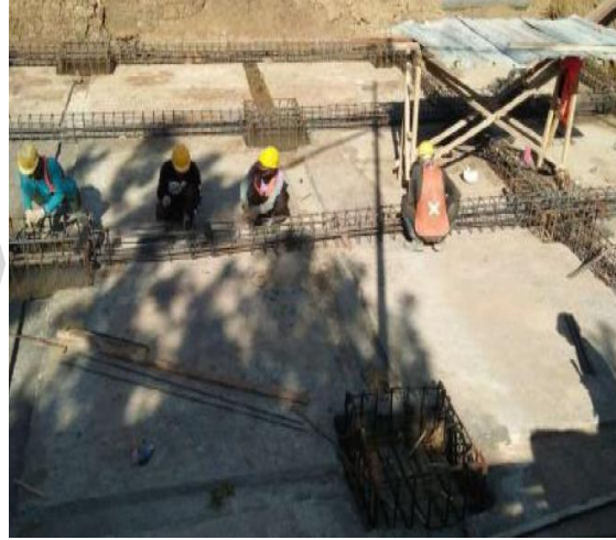
Foundation work of the plant
