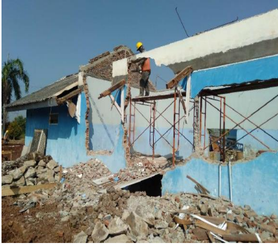
Demolition of existing facilities
